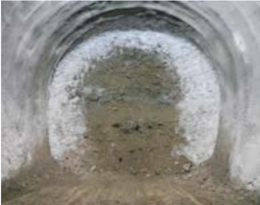
Above: AGF excavation
